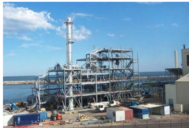
Esterfip-H unit under construction in Sète, France.
