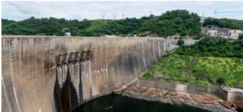
Large-scale dam projects, such as the Kariba Dam, create large reservoirs for water storage.
